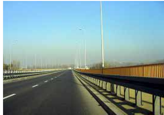
Figure 4 Road barriers: concrete barrier (Zakopiańska) and steel barrier. (source: ITC, Bulgaria and the Cracow University of Technology)
